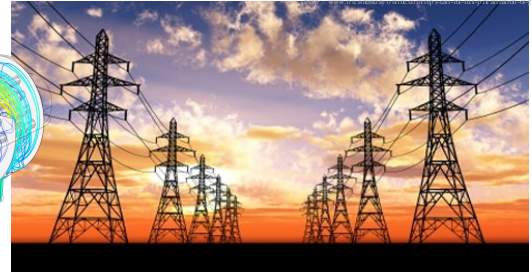
Power generation sector
